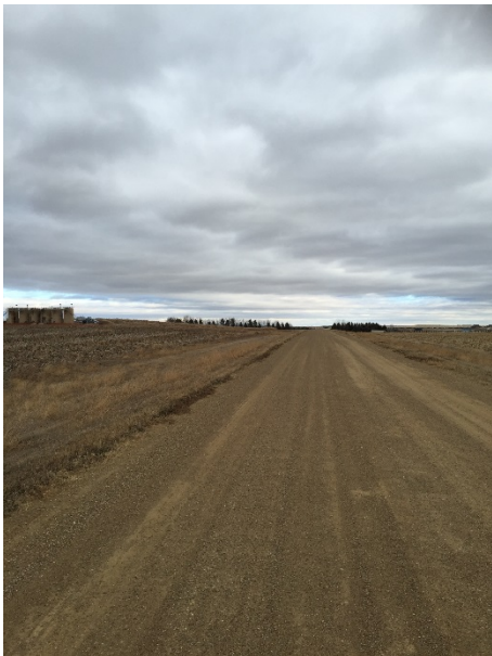
FIGURE 2-VIEW OF 41 ST SW
