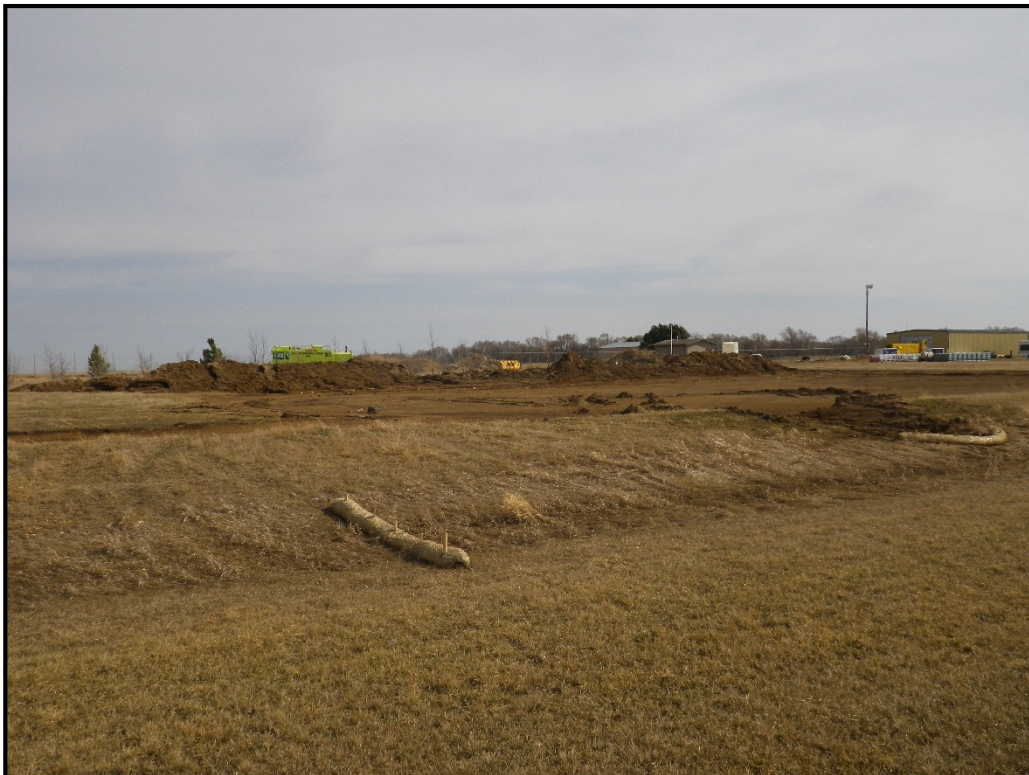
Figure 24: Disturbed portion of APE to the east of the airport hangers, view to the north.
