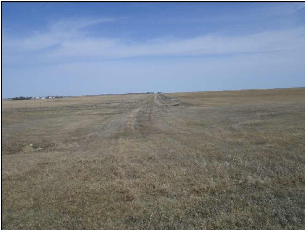
Figure 15: View of north segment of raised road bed from airport runway, view to the north.
