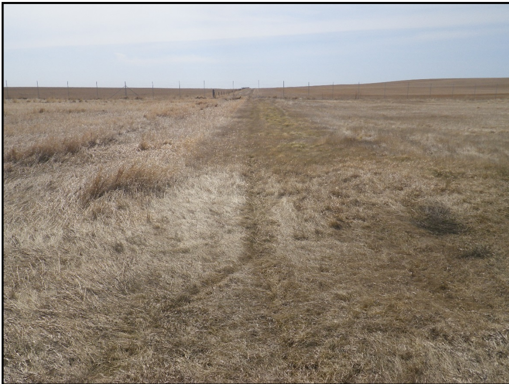
Figure 17: View of south segment of raised road bed from airport runway, view to the south.
